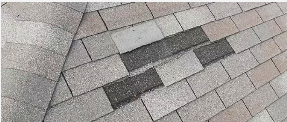
MISSING SHINGLES
